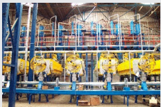
16,000 t/y litharge plant (UK)
